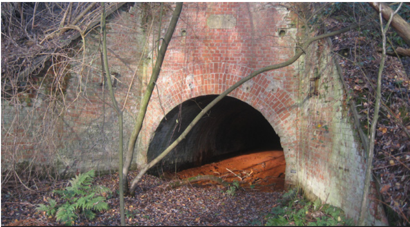
Tunnel 36, foto PA
